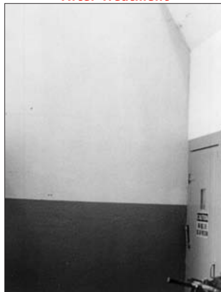
Treatment was made from the negative side against the hydrostatic weeping.
